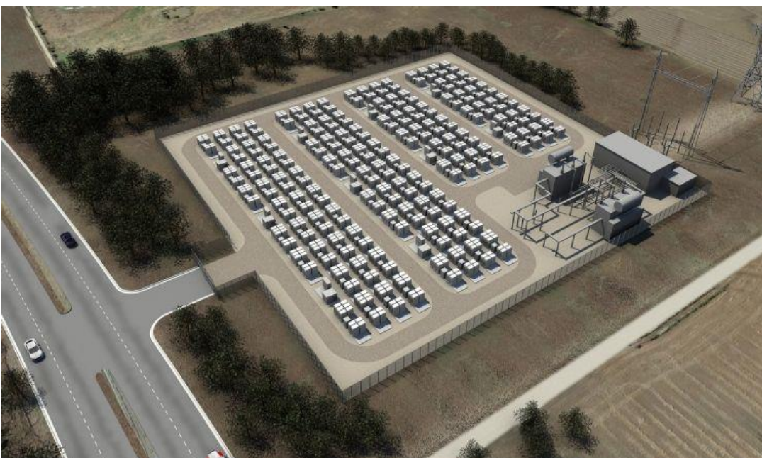
FIGURE 8-6 SOLARCITY'S TESLA BATTERY STORAGE FACILITY, HAWAII
