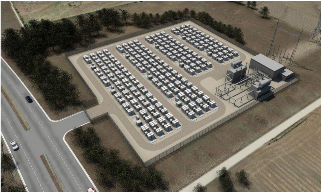
FIGURE 8-6 SOLARCITY'S TESLA BATTERY STORAGE FACILITY, HAWAII
