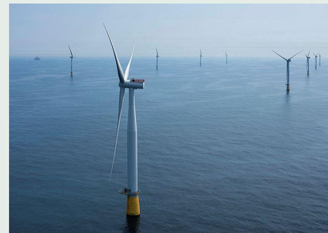
In 2023, the 88 MW Hywind Tampen floating project reached COD. It consists of 11 turbines and is now the largest floating offshore wind project globally. Source: Equinor
