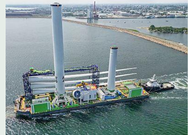
In 2023, the first of 62 GE Haliade 13 MW turbines were installed using feeder barges at the 800 MW Vineyard Wind 1 project in the U.S. Source: BargeMaster.
