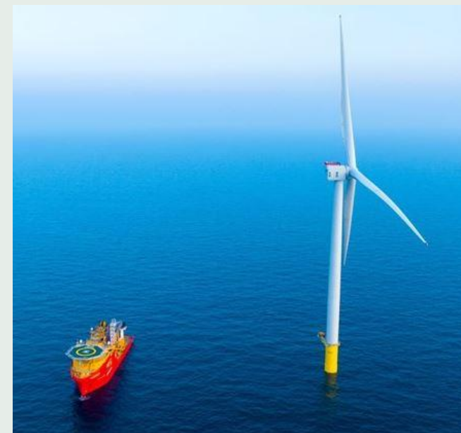
In 2023, first power was achieved at Dogger Bank, the world's largest offshore wind project. Source: SSE
