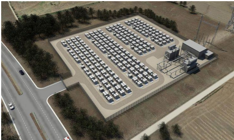
FIGURE 8-6 SOLARCITY'S TESLA BATTERY STORAGE FACILITY, HAWAII
